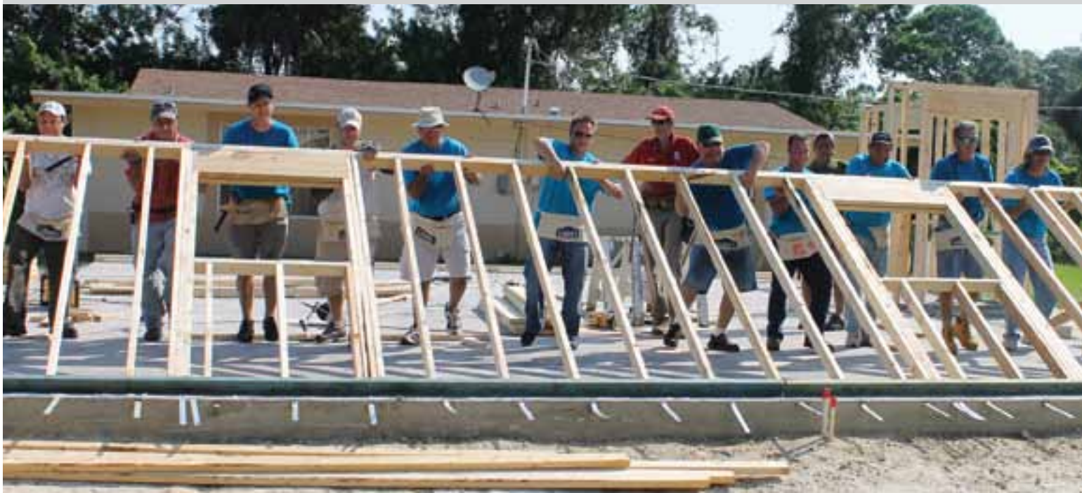
Volunteers from Naples Yacht Club raise walls on a new Habitat home.
